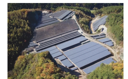
Solar Power on Samcheok Mine Site
