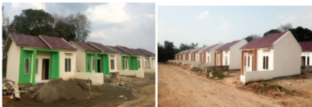
Gria Pali Residence at Pali - Palembang, Indonesia
