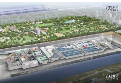
Changes in Bakdal sewage treatment plant
