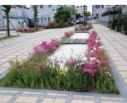
Infiltration ditch
