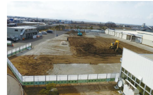
Ground concrete reused as gravel (white areas) (September–October 2018)
