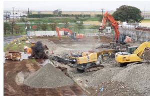
Concrete is ground up by a Galapagos crusher (September–October 2018)
