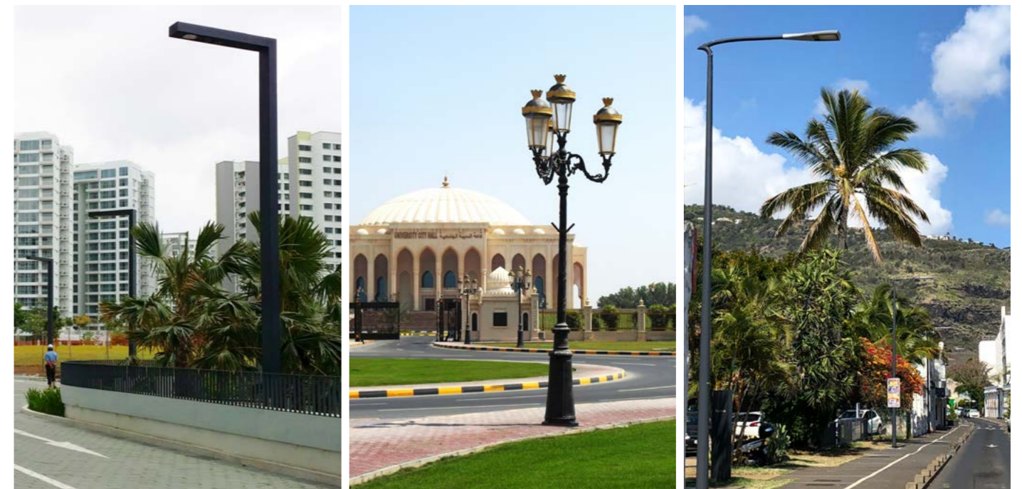
Ragni light fixtures installed in Singapore (left), Qatar (middle), and Réunion Island.
