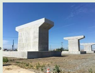
Piers for the Chinju Bridge in Ishinomaki City, Miyagi Prefecture
