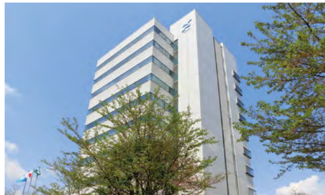
Backup facility (Kita-ku, Tokyo)
