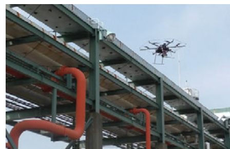
Inspections using drones
