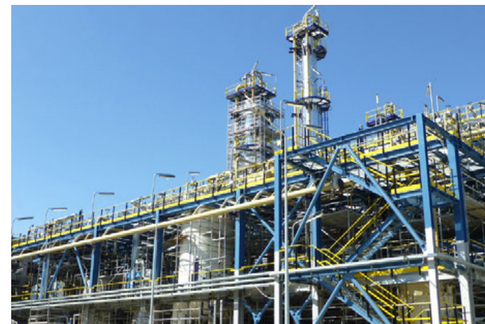
The SSBR Hungary Plant (completed in April 2019)
