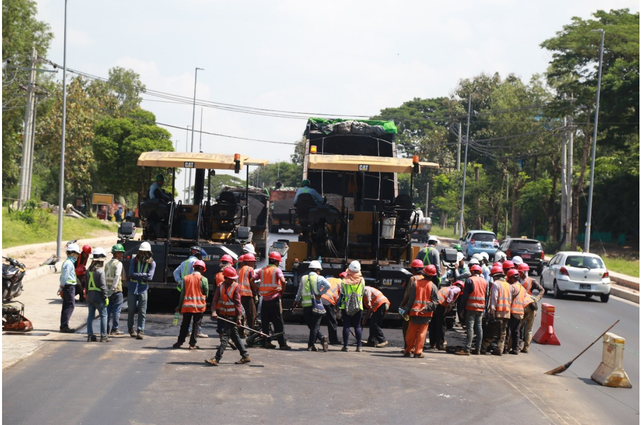
Figure: Construction of the AC Plasterers of Thanlyin-Thilawa Access Road Project
