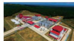
Unifuji is located on United Plantation's vast oil palm farm.
