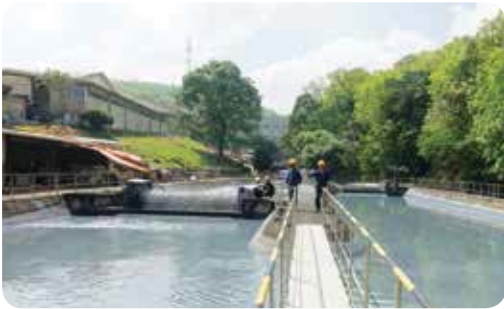
Effluent treatment plant
