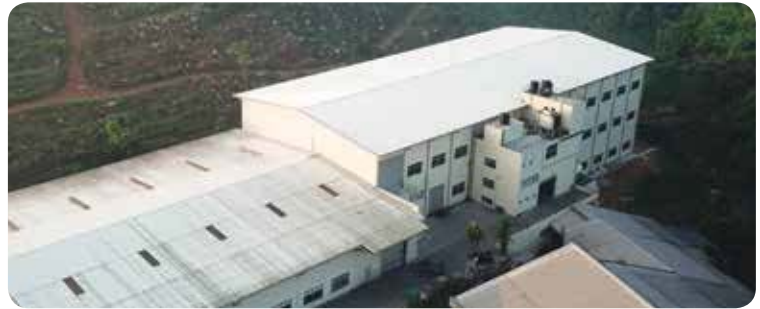
Establishment of the new knitting building
