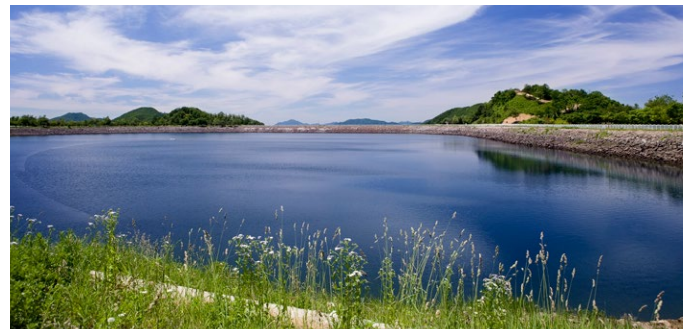
▲ the higher-elevation reservoir of Cheongpyeong Pumped-Storage Power Plant
