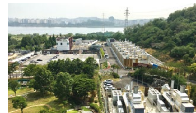
▲ Noeul Fuel Cell Power Generation Plant
