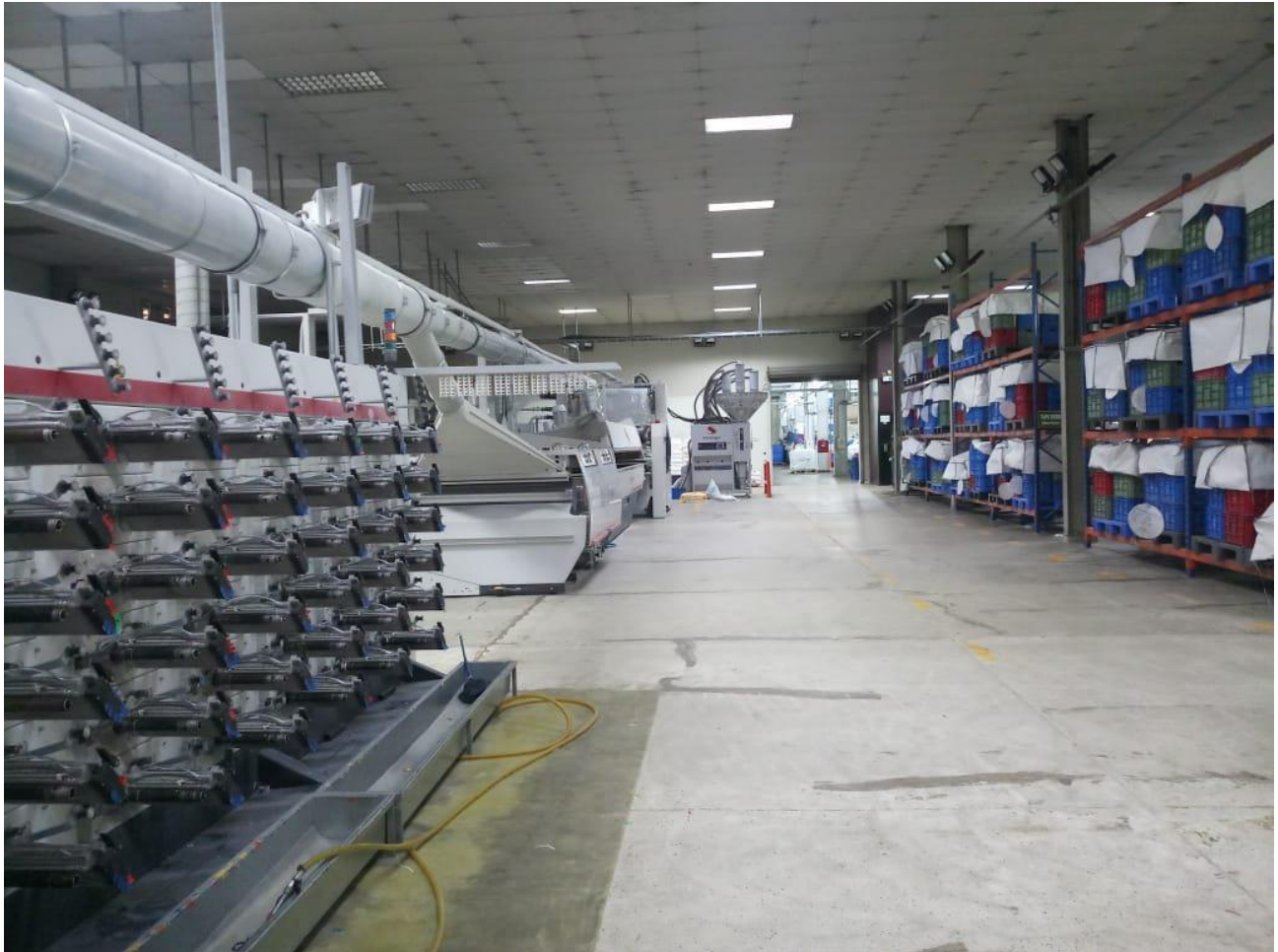
Racks placed to reduce sound.
