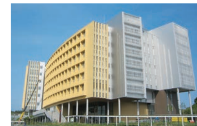
Agricultural Research Building, Ito Campus, Kyushu University (air conditioning installation)
