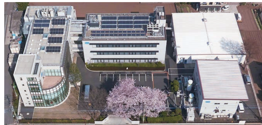
Aerial view of our Technical Research Laboratory in Miyoshimachi, Iruma-gun, Saitama Prefecture
