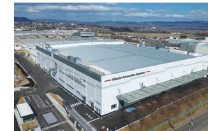
R&D Bldg. and Factory No. 5, Fukushima Plant Hitachi Automotive Systems (air conditioning and plumbing installations)
