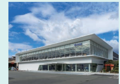
Installation example ③ Teral Inc. New ZEB Office
