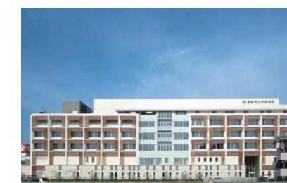
Kurashiki Municipal Hospital, Kojima (air conditioning and plumbing installations)
