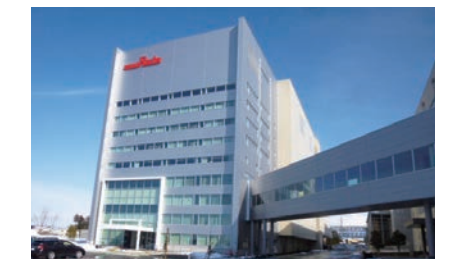
Building D, Toyama Murata Manufacturing (air conditioning and plumbing installations)
