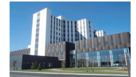
Obihiro Kosei Hospital (plumbing installation)
