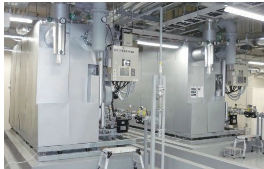
Gas-fired absorption-type cold/hot water supplier
