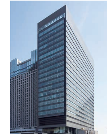
Namba SkyO (electrical, air conditioning and plumbing installations)
