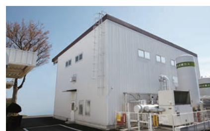
Supercritical CO 2 cleaning plant
