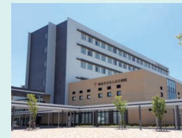
Installation example ① Takamatsu Municipal Hospital
