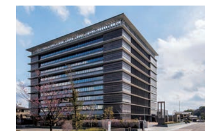
Wakayama Regional Joint Government Building (air conditioning and plumbing installations)
