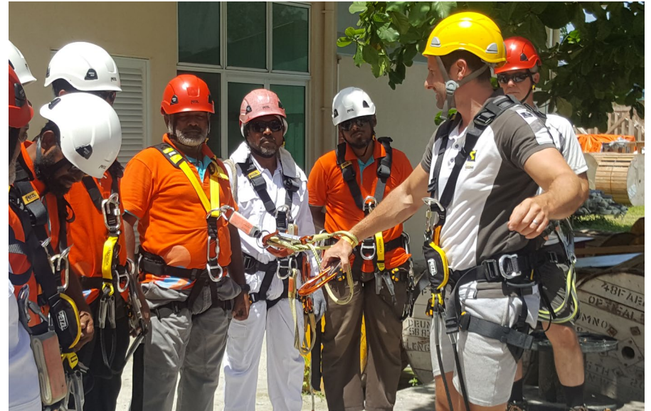
Basic rigging with tower climbing training was carried out for all newly joined riggers.
