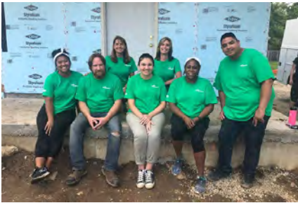
Helping to repair homes for low-income people through Habitat for Humanity (Systemex America)
