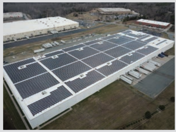
Solar panel installation at Lenovo Whitsett, North Carolina facility - March 2019.
