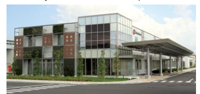
Daiwa KOMFORT (our Ryugasaki Plant Office Building)
