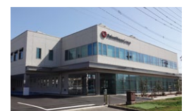
Electricity self-sufficient building (Daiwa House Saga Building)
