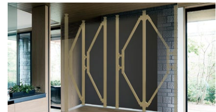
Newly developed load-bearing wall “Kyurek”
