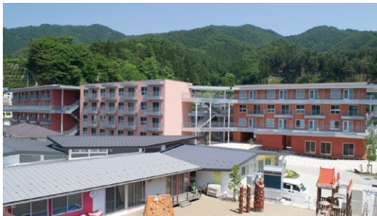
Tenjin Restored Housing
