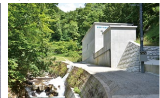
Hydroelectric Power Plant No.1
