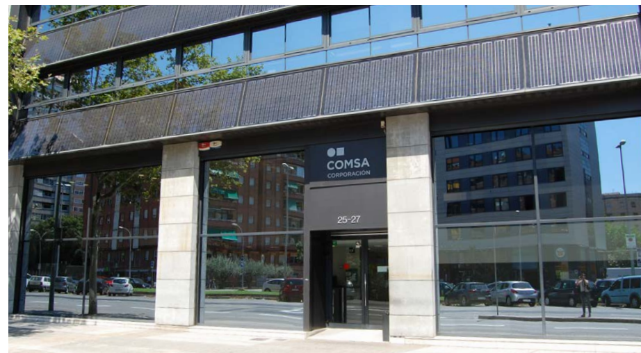
ISO 50001 certification of the office building at Av. Roma, 25 in Barcelona (Spain)
