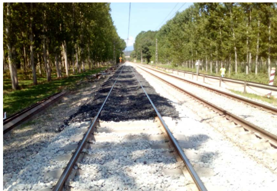
Application of Neoballast in a test section, Caldes de Malavella (Spain)
