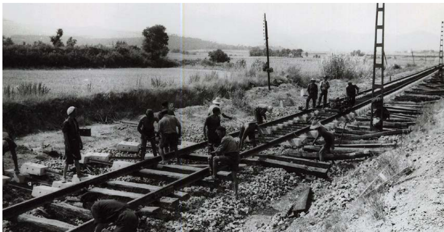
Track renovation work between Celrá and Figueres, 1961 (Spain)
