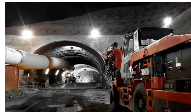
Amagá Tunnel on the Pacifico 1 motorway (Colombia)
