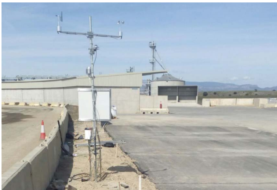
Test section with Albepav sustainable asphalt, Balaguer (Spain)
