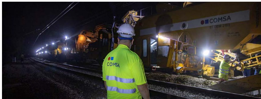
Track renovation in Maçanet de la Selva-Caldes de Malavella (Spain)
