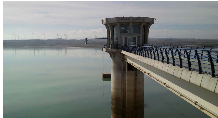
La Serena reservoir intake tower, Badajoz (Spain)
