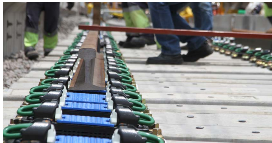
Maintenance of Line A of the Mexico City Metro (Mexico)
