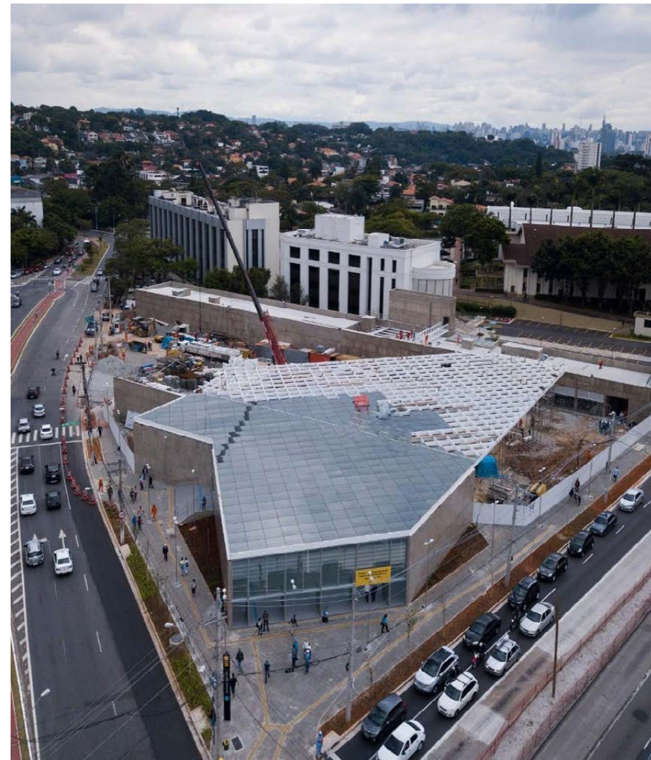
Second phase of Line 4 of the Sao Paulo Metro (Brazil)
