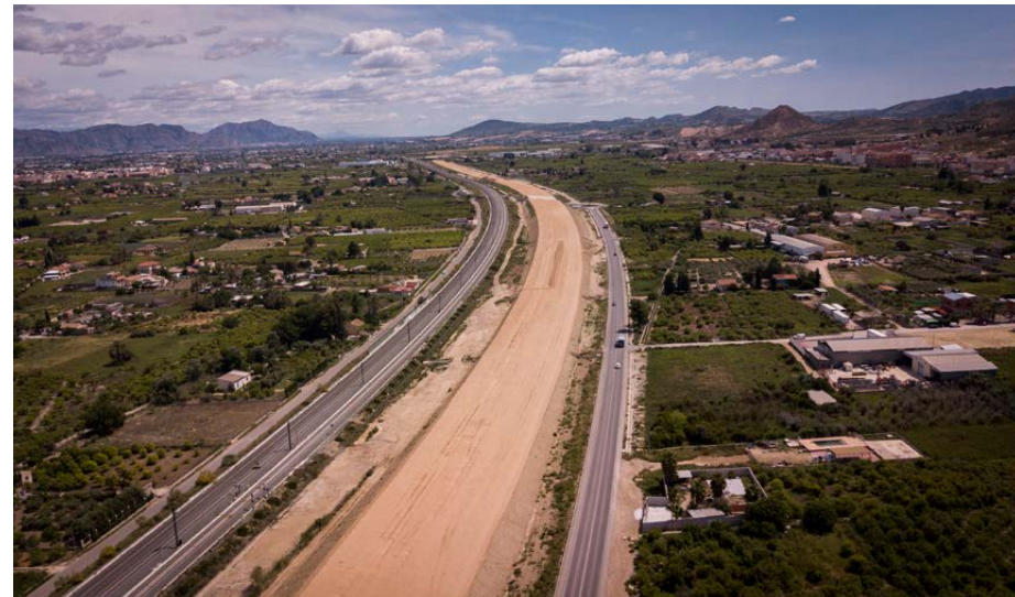
Construction of the Reguerón Motorway, Murcia (Spain)
