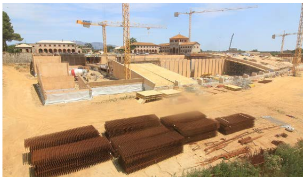
Construction of the Perelada Group winery, Girona (Spain)
