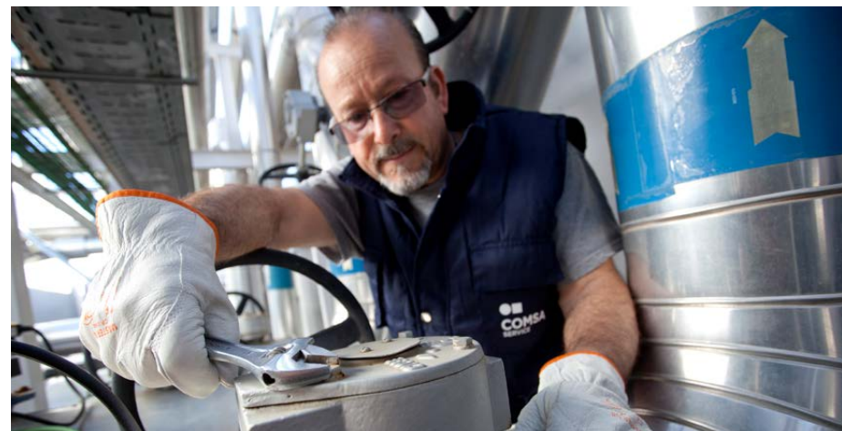
Improving energy efficiency and maintenance in buildings (Spain)
