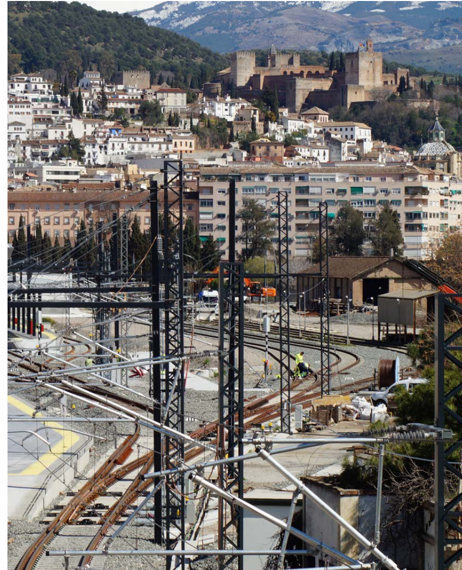
Adaptation of the Granada station for high-speed trains (Spain)
