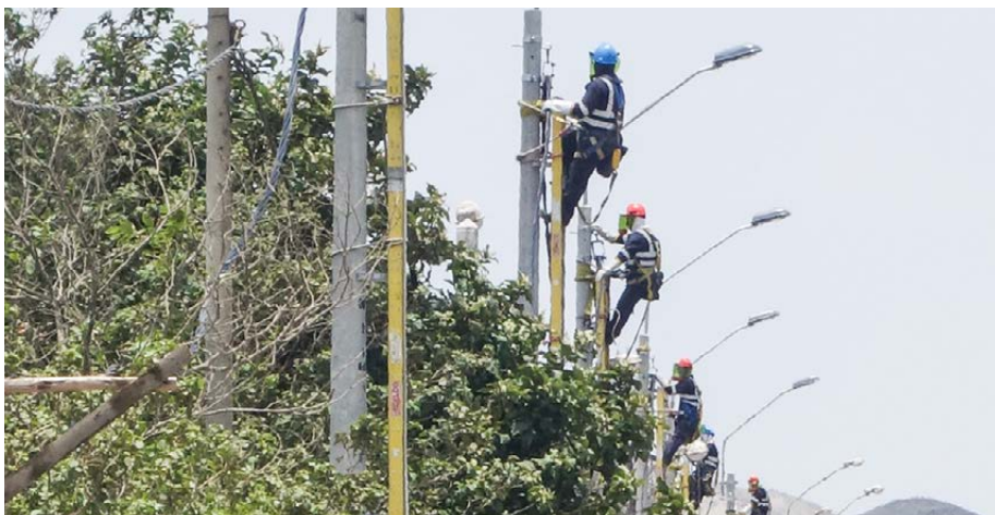
High, medium and low voltage electrical works in Lima (Peru)
