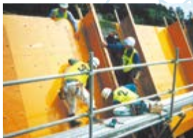
High-strength aramid fiber serves as a reinforcement material at public works sites
