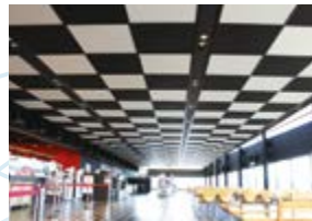
The ultra-lightweight ceiling material Kal-ten helps to mitigate hazards during earthquakes
