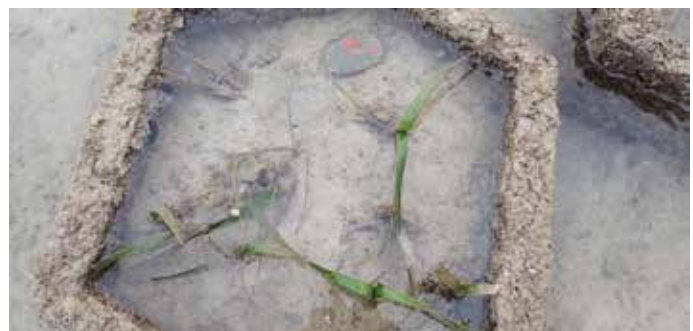
Seagrass contained in hexagonal hollow concrete blocks to minimise soil loss caused by strong currents and wave attrition
