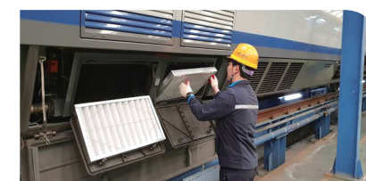
Replacing Filters of Air-Conditioning Systems
