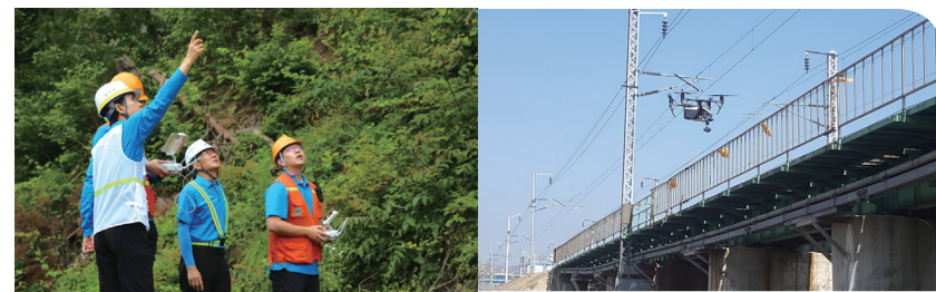
Inspecting Railway Facilities by Utilizing Drones
