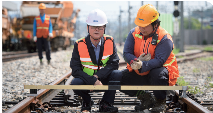
Field Inspection at Gangneung Station
