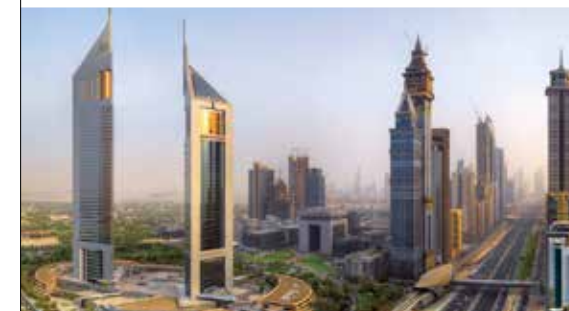
2011 Dubai Metro Project
