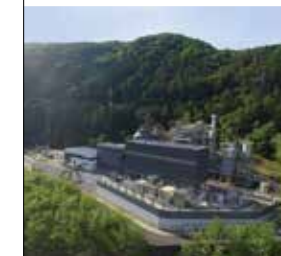
2018 Otsuki Biomass Power Plant
