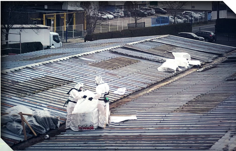
Asbestos removal on the roof of the OMERIN division principale building
