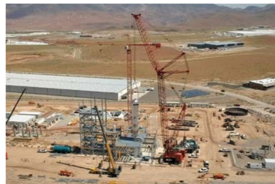
Fulcrum's SAF plant under construction in Nevada (May 2019)
