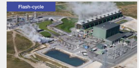
Nga Awa Purua Geothermal Power Station (140 MW generation capacity, New Zealand)
