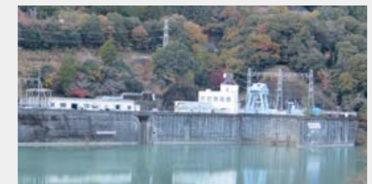
Akiha No. 1 Power Station of Electric Power Development Co., Ltd. (47.2 MW, Shizuoka Prefecture, Japan)
