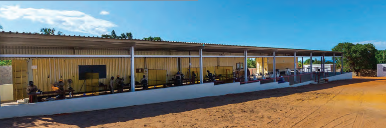
Training centre in Inhassoro, Inhambane Province, Mozambique
