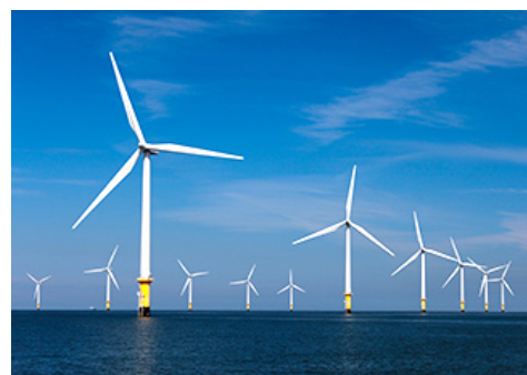
Butendiek Wind Power Plant
