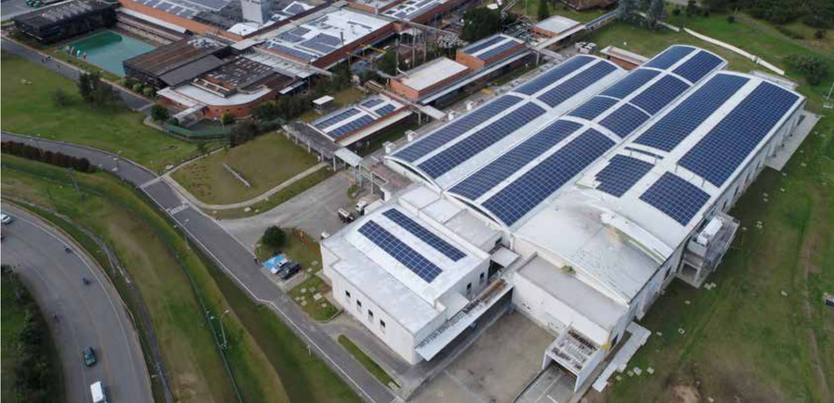
Solar panel roofs of the Chocolates Business facilities in Rionegro, Colombia.
