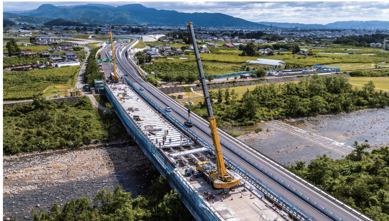
Expressway Renewal Project (TOHOKU EXPWY between Fukushima-Nishi IC and Fukushima JCT)
