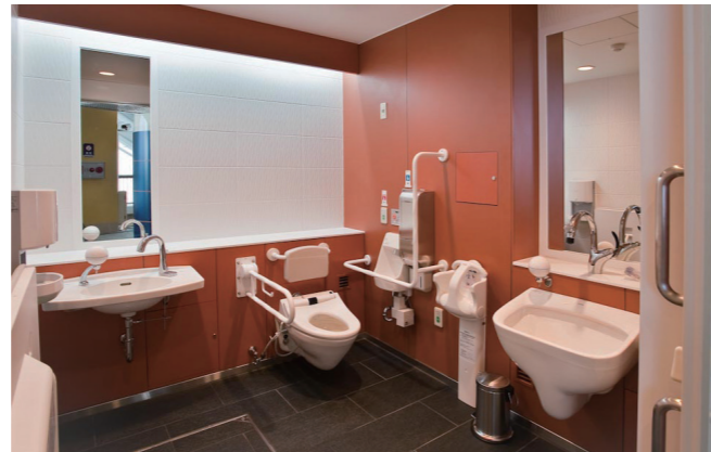
Multifunctional restroom (universal toilet)
