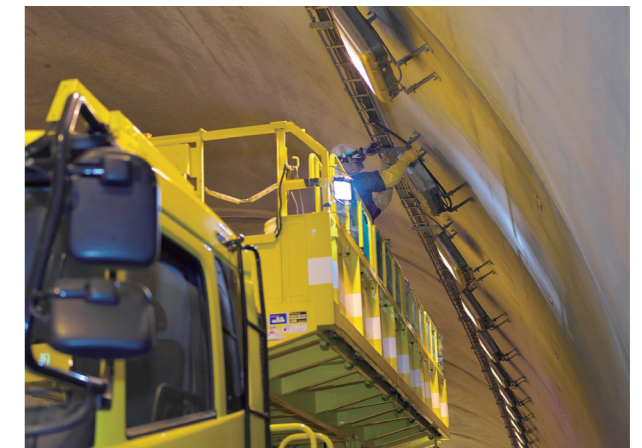
Cleaning the lights in a tunnel
