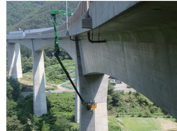
Hammering test inspection on bridge
