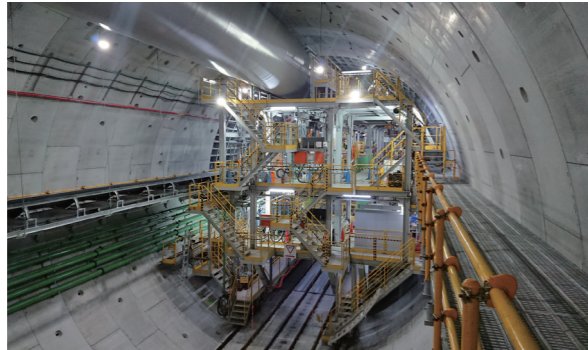
Tunnel construction using shield machine
