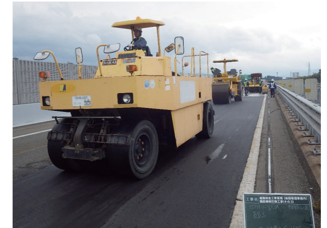
Repairing road surface
