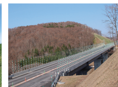
Installation of bird flight guiding poles
