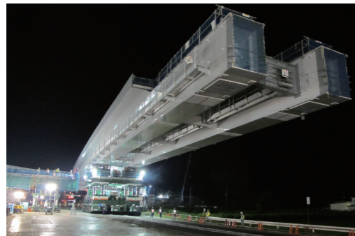
Consolidated viaduct construction using a multi-axle truck
