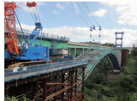
Cable erection work
