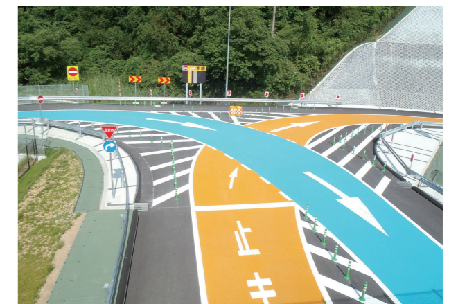
Measure to prevent wrong-way driving at flat intersection of flat Y-shaped IC
