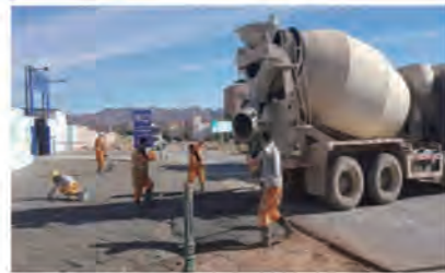
为业主SSC公司修路 Building a road for the Owner SSC
