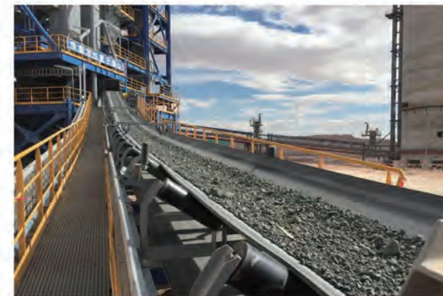
中材建设阿尔及利亚BIKSRA项目水泥调配站入料 Cement mixing station feeding in Algeria BIKSRA project of CBMI
