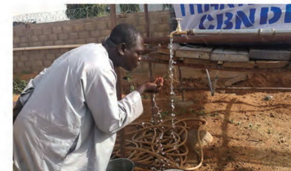
尼日利亚SOKOTO项目为当地村民提供生活用水 Nigeria SOKOTO Project Department provided domestic water for local villagers
