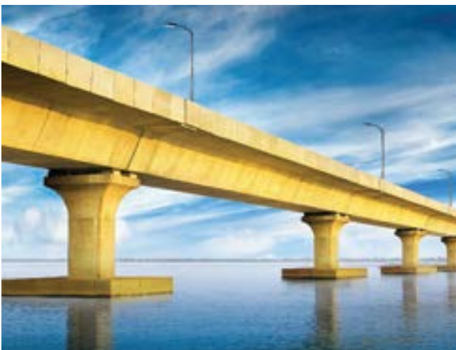
Dhola-Sadiya Bridge, Arunachal Pradesh
