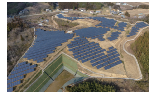
Solar power plant in Tome, Miyagi Prefecture
