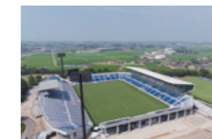
Kumagaya Rugby Stadium in Saitama Prefecture
