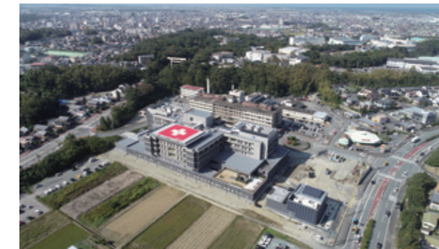
Ise Municipal General Hospital in Mie Prefecture
