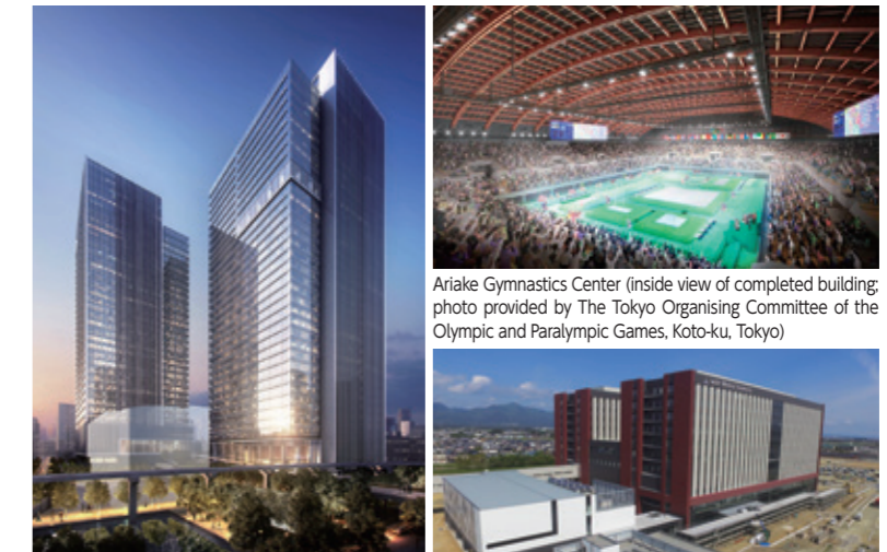
msb Tamachi Station Tower North (Completed perspective (right), Minato-ku, Tokyo)
