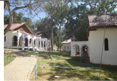
Villas under construction
