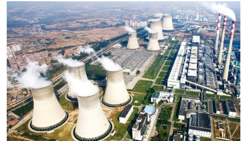
8 units of Datang Yangcheng Power Generation Company complete ultra-low emission transformation.
