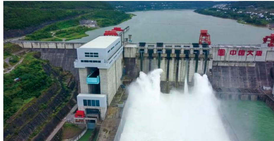
Datang Tingzikou Hydropower Station
