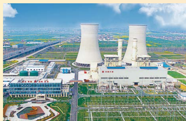
Datang Taizhou Thermal Power Co Ltd, the best gas turbine project of CDT in terms of costs and the first smart power plant in China
