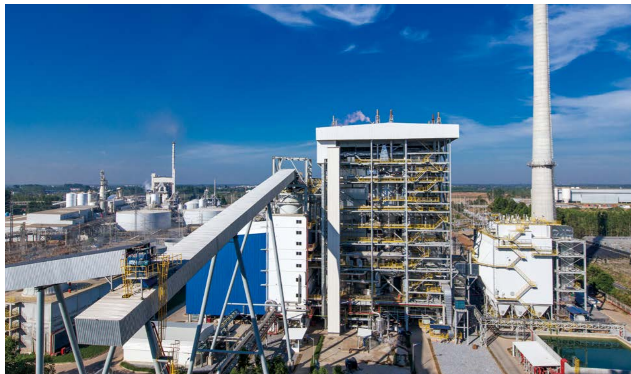
The general contracting projects of the NPP5A and NPP9 biomass power plants in Thailand are the "bellwethers" of CDT's overseas development. The NPP9 project is the largest biomass power station in Asia, fully demonstrating our strength in undertaking contracted projects overseas.
