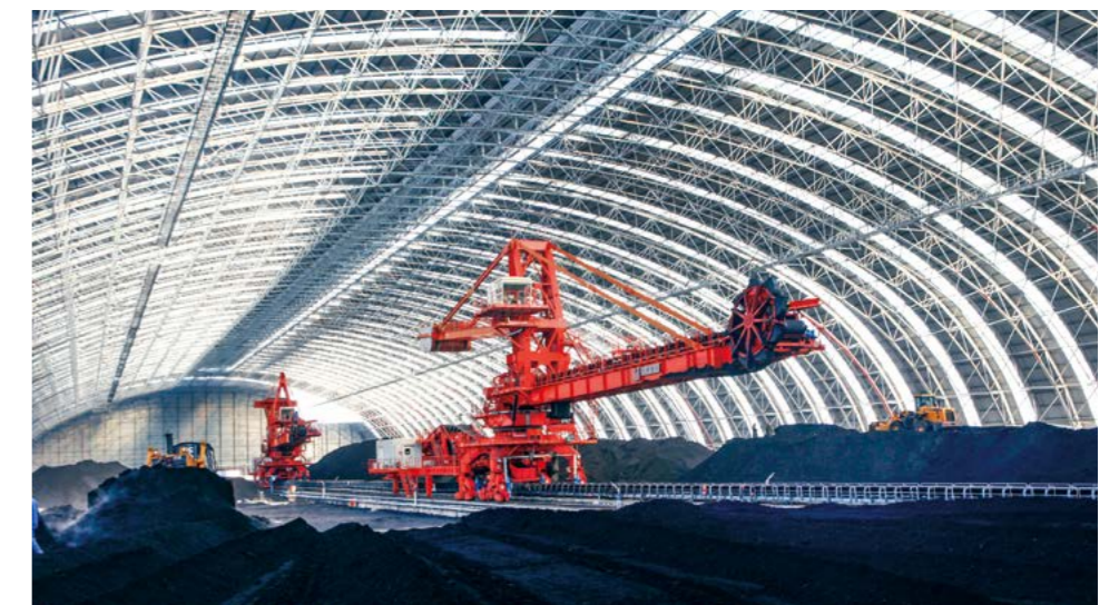
The closed coal yard of Datang Binzhou Power Generation Company
