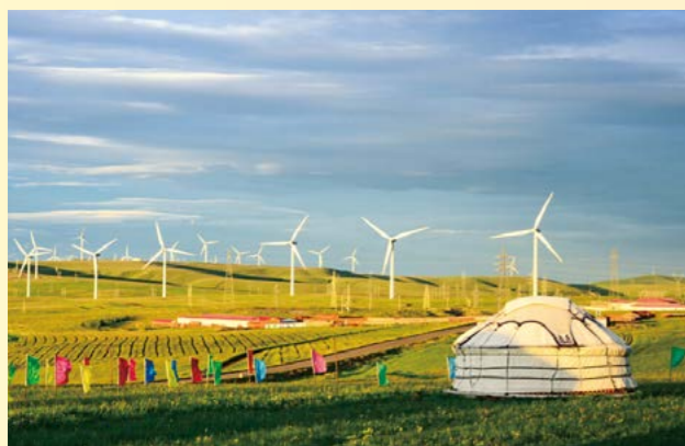
Datang Chifeng Hanshan Wind Power Company, the best wind power project of CDT in terms of costs and profits
