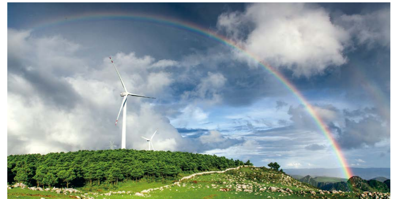
The first top-quality wind power project of CDT - Datang Qiubei Wind Farm
