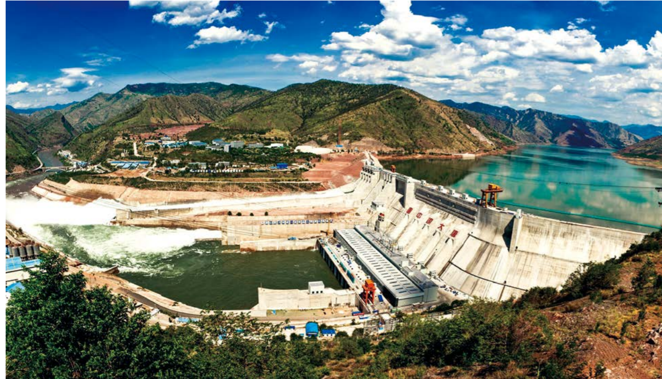
The Grade 1 hydropower project for power production safety standardization - Datang Guanyinyan Hydropower Station
