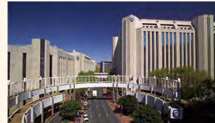
Buildings of Standard Bank Group
