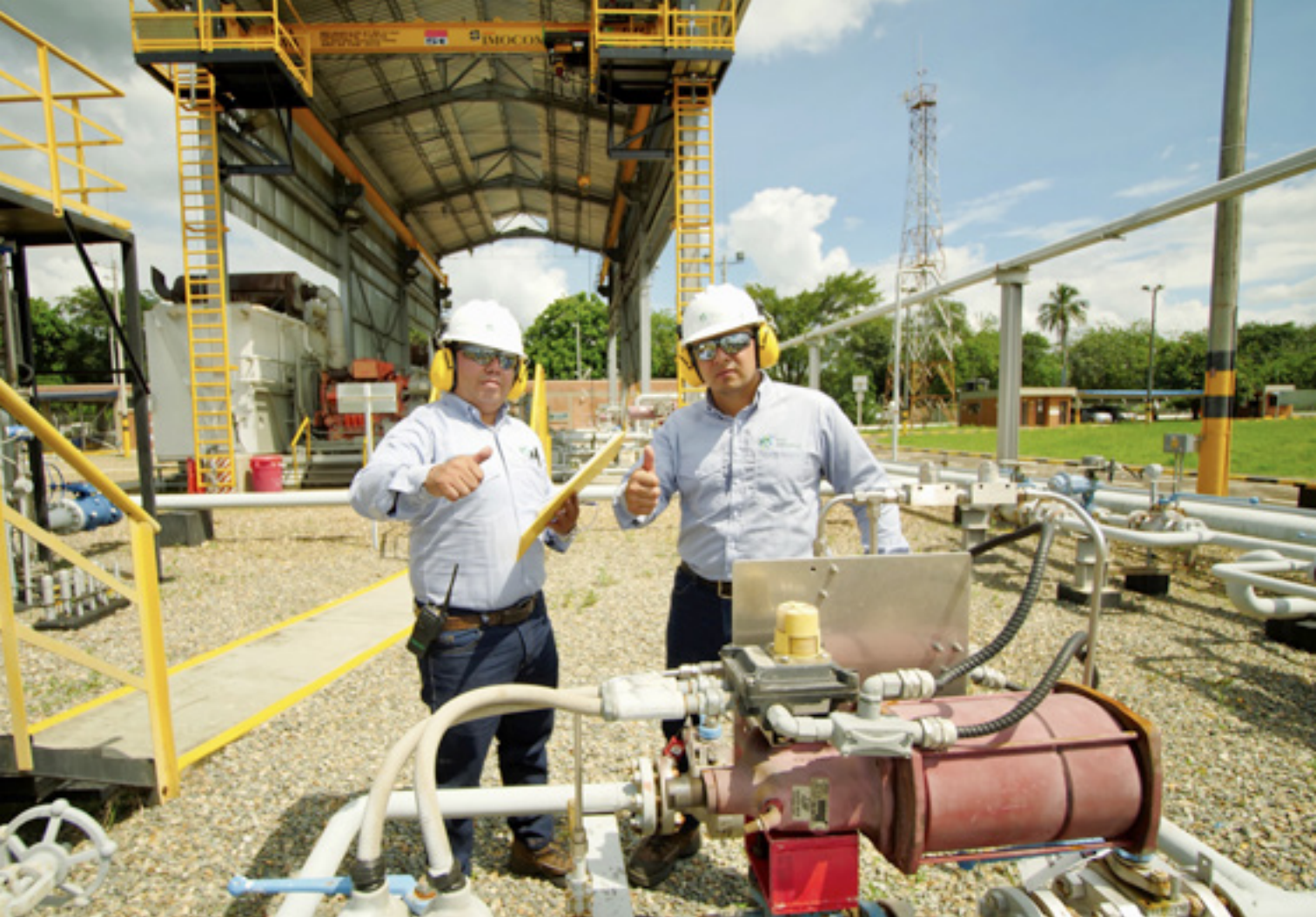
TGI engineers at the Mariquita Station, Tolima
