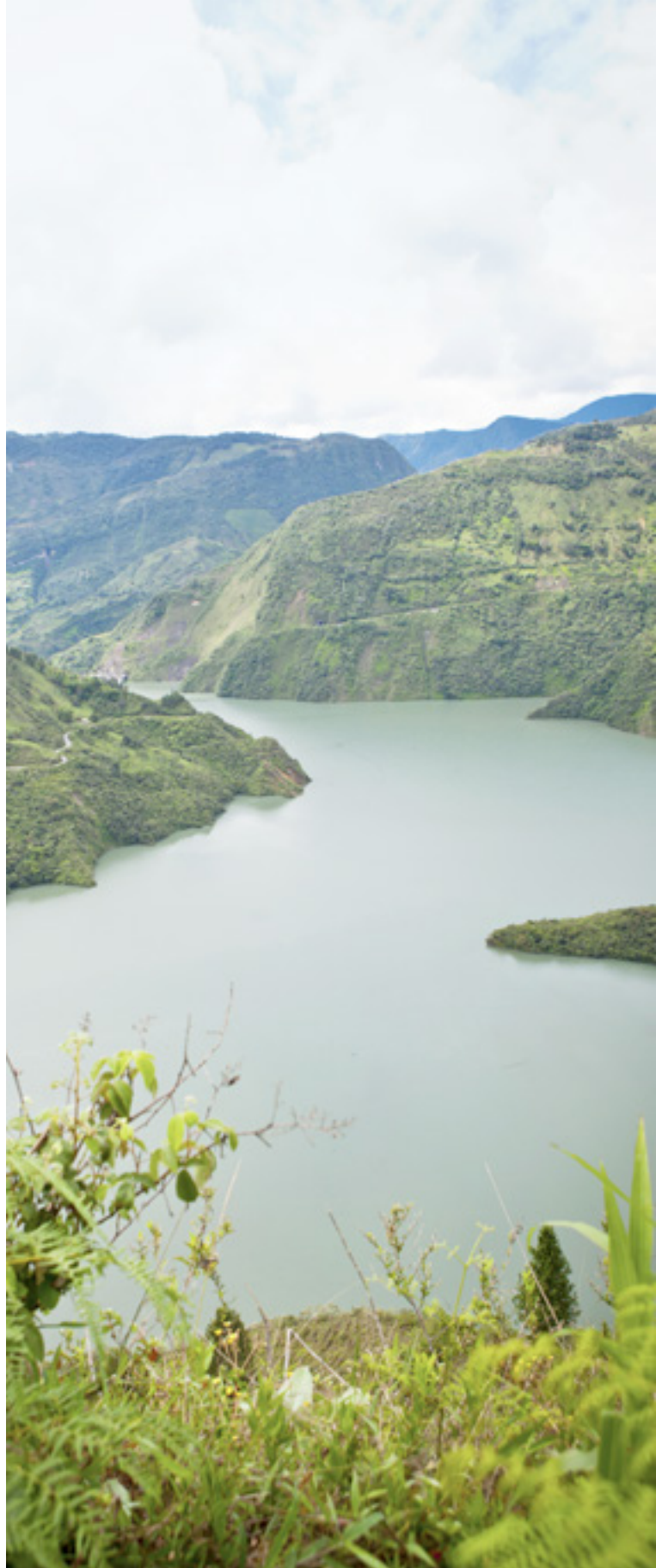
Guavio Reservoir, which feeds the hydroelectric power plant with the same name. Grupo Energía Bogotá Project in Cundinamarca
