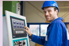
For facility operation and security control
