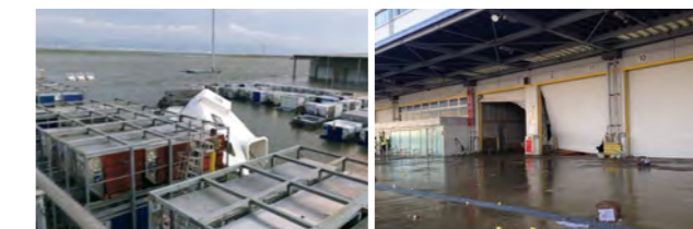
Left: Flooded cargo operations area at Kansai International Airport. Cargo containers were submerged and high winds damaged the roofs of boarding ramp vehicles. Right: Import cargo shed shutters were damaged by high winds, while heavy rain and storm surge caused flooding.
