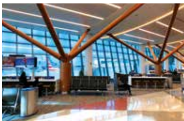
The Boston Logan Airport installation, Electrochromic windows by View, Inc. with NSG Group TEC™ glass
