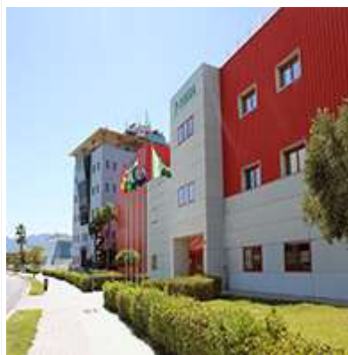
DEKRA Headquarters Building Málaga – Spain
