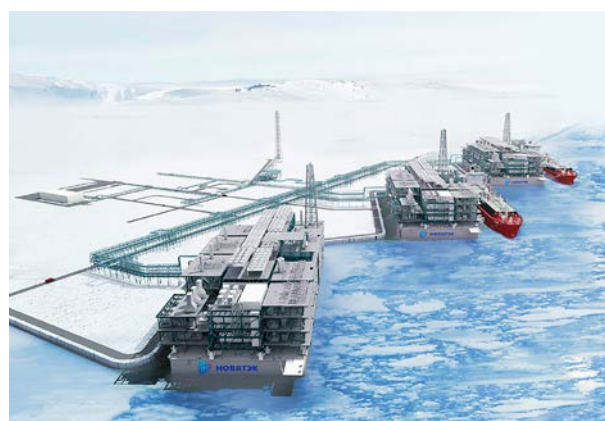
Liquefaction facility mounted on a concrete structure stabilized on the sea bed
