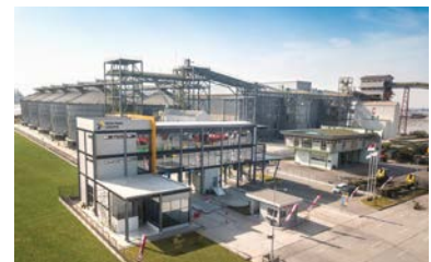
FKSFA's grain import facility
