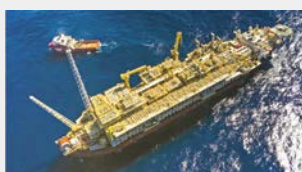
FPSO operating in Brazil ©MODEC, Inc.
