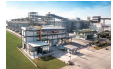
FKSFA's grain import facility
