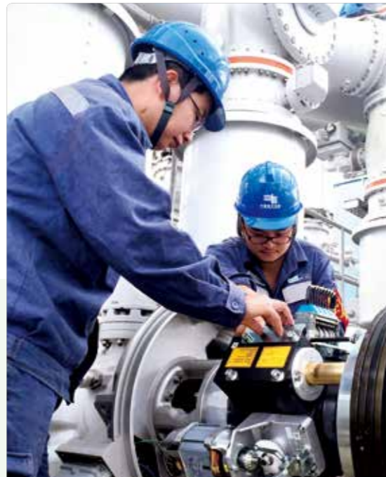
Ultra-high voltage company performing substation equipment maintenance.
