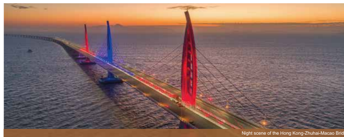
Night scene of the Hong Kong-Zhuhai-Macao Bridge
