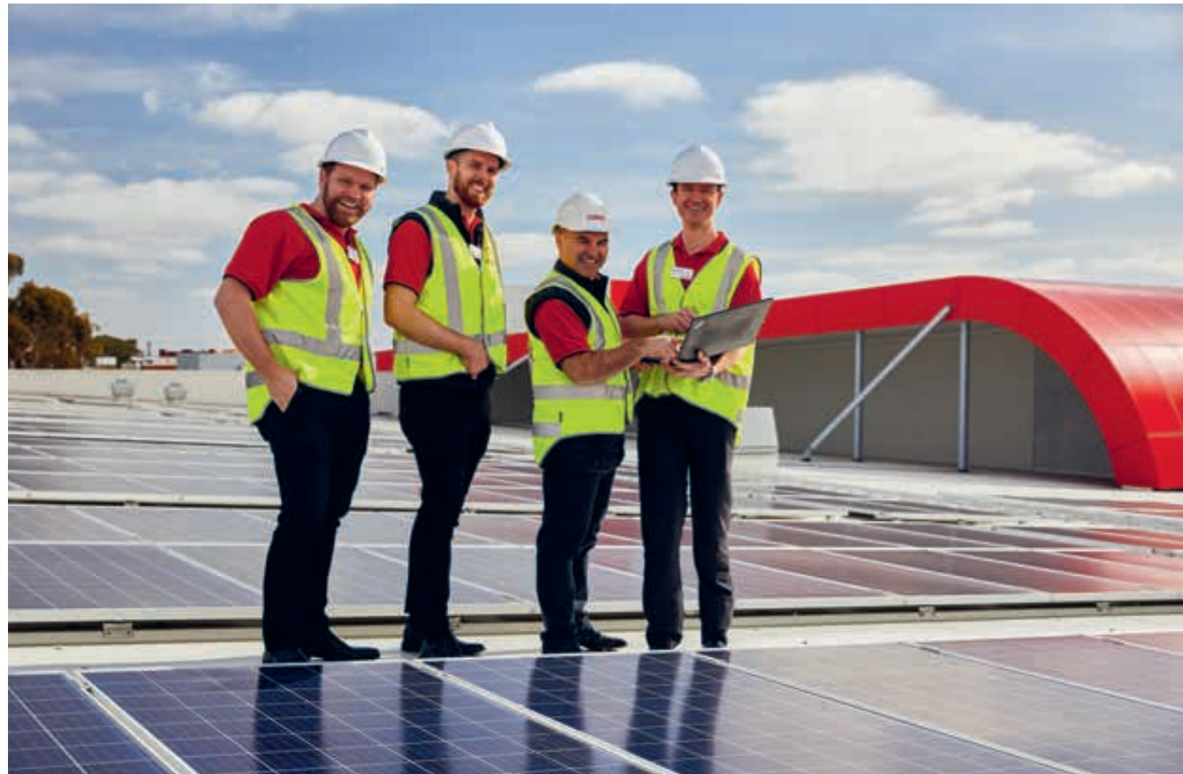
Coles team members Andrew, Alex, George and Andrew (left to right) inspect solar panels on the roof of Coles' supermarket at Drysdale, Victoria. By the end of FY19, Coles had 30 supermarkets connected to solar power.
