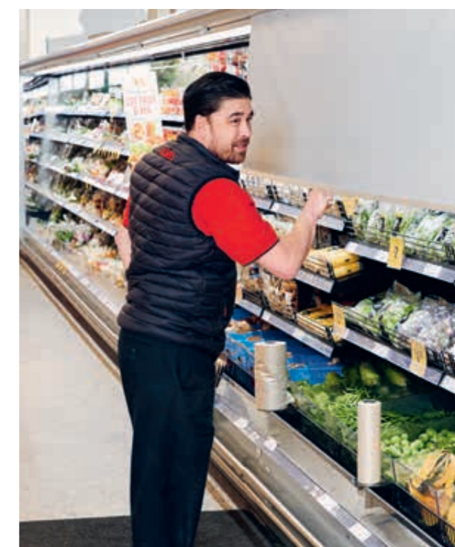
Fresh Produce Manager David from Coles Victoria Gardens, Richmond, Victoria lowering night blinds used on refrigeration units to reduce energy consumption.
