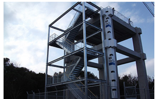
Evacuation tower in Nobeoka, Miyazaki Prefecture
