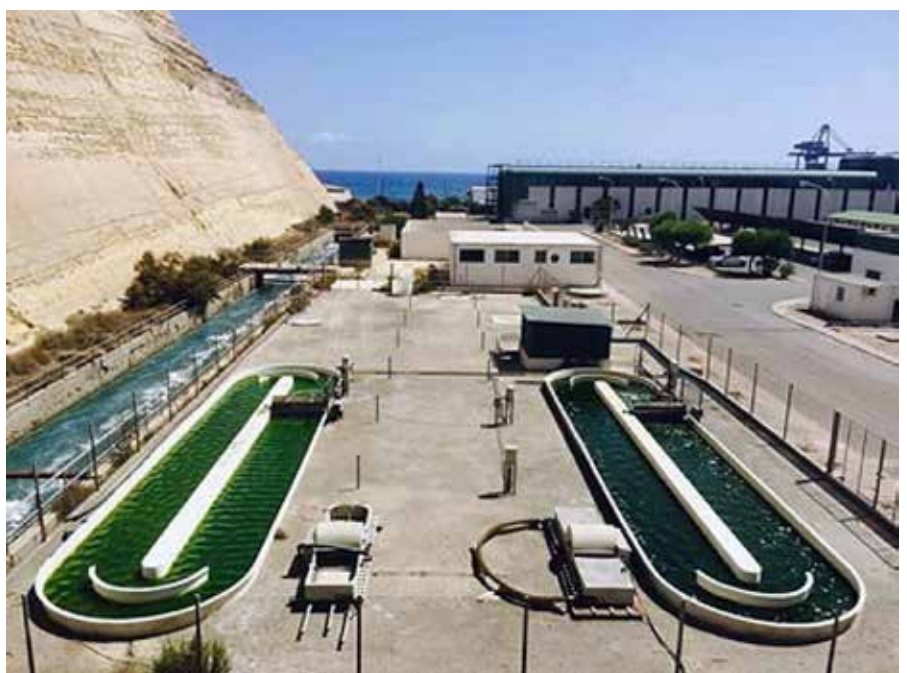
Microalgae pilot facility at the Litoral Thermal Power Plant in Almería.
