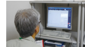
Demand monitoring equipment at the head office building
