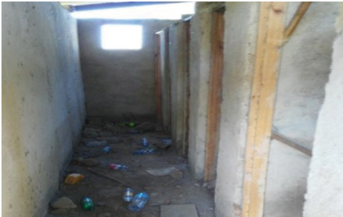
Mbeya - Itiji primary school cloak room (before)
