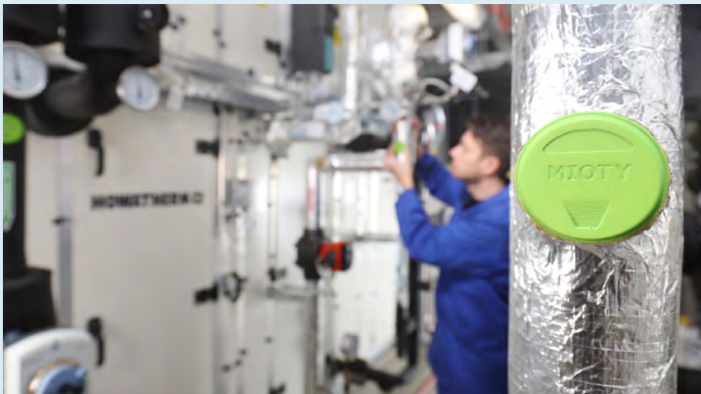
Robust systems are used to transmit sensor data and control information across network infrastructures. MIOTY, a miniature IoT system developed by Fraunhofer IIS, sets new standards in the field of wireless data transmission.
