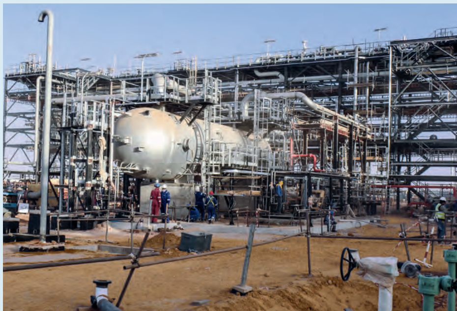
As the result of an audit, in Reggane, DEA developed an environmental and social action plan (ESAP) in cooperation with an external consulting agency.
